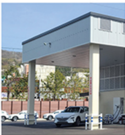
Ulsan Hyundai Motors Charging Station
