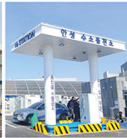
Anseong Charging Station
