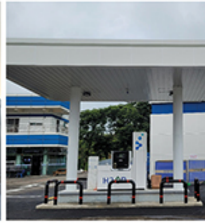
Dangjin Charging Station
