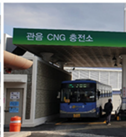
Daegu Gwaneum Charging Station
