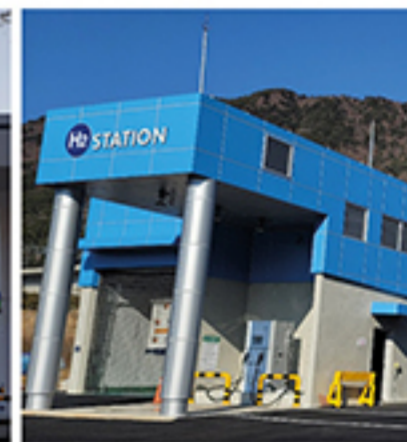
Changwon Sarim Charging Station
