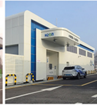
Suwon Gwanggyo Service Area Charging Station
