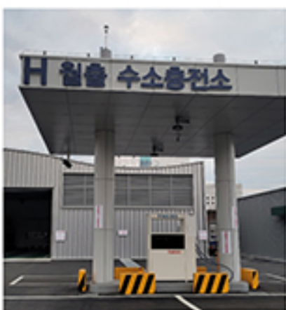
Gwangju Wolchul Charging Station
