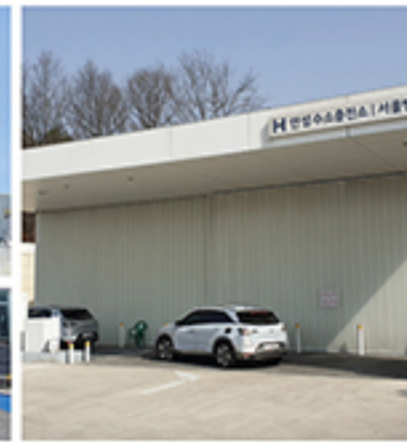
Anseong Service Area Charging Station
