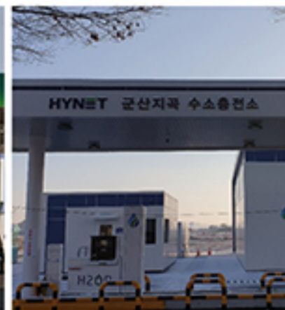
Gunsan Jigok Charging Station
