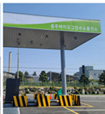
Chungju Charging Station
