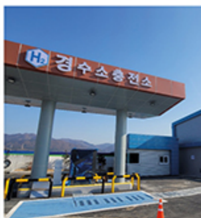
Ulsan Changpyeong Charging Station
