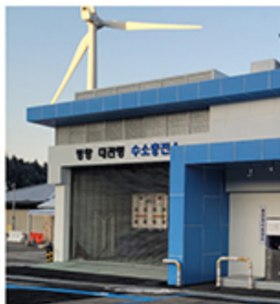
Daegwanryeong Charging Station
