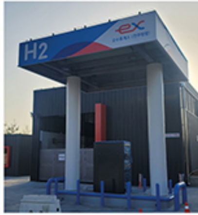
Osu Charging Station
