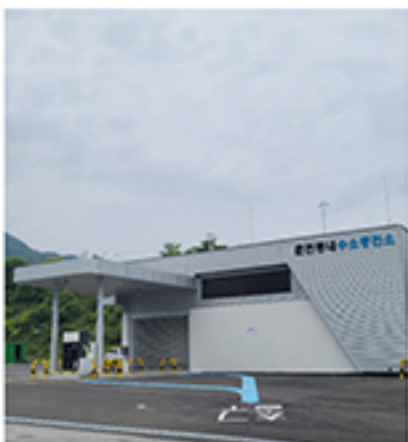
Chuncheon Charging Station
